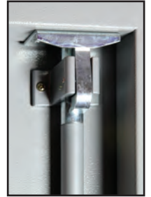
Door head frame pre-drilled to accept top trip and top shoot
