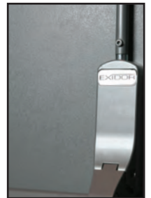
Door leaf is prepared for the Exidor 294 panic bolt
